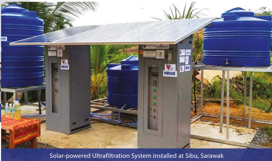
Solar-powered Ultrafiltration System installed at Sibu, Sarawak
